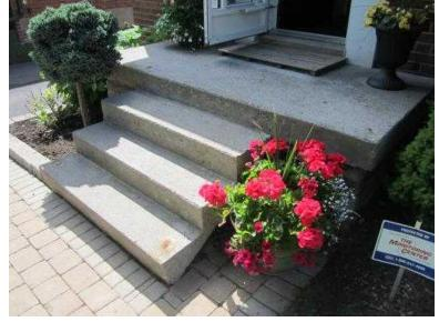
3. Marginal Porch: Concrete: Missing handrails (liability, safety issue). Moisture damage to side surface - monitor
