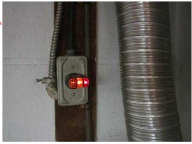
7. Acceptable Dryer Vent: Metal flex: Flex duct restricts air flow and traps more lint than smooth walled rigid
