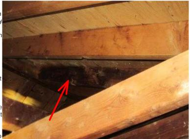
7. Acceptable, Improve Insulation: Loose fill fibreglass, Fiberglass batts: Insulate and weatherstrip hatch to minimize heat loss or condensation buildup in attic from warm heated air entering the attic and cooling, R24-36 approximate, because insulation levels are not even, but overall this is an acceptable level of insulation. Consider improvements if necessary after living through the first winter.
